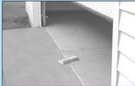
FIG. 6-5 2 x 4 under center of door opening.
