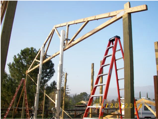
Above two Genie Superlifts are used to raise a truss pair.
