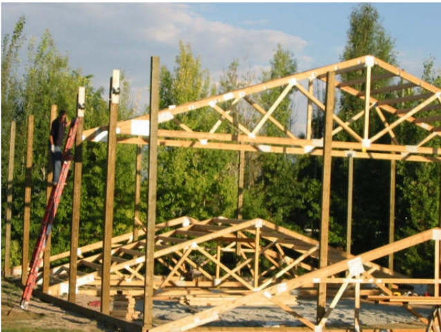
Two truss pairs being “cranked” into place with winch boxes
