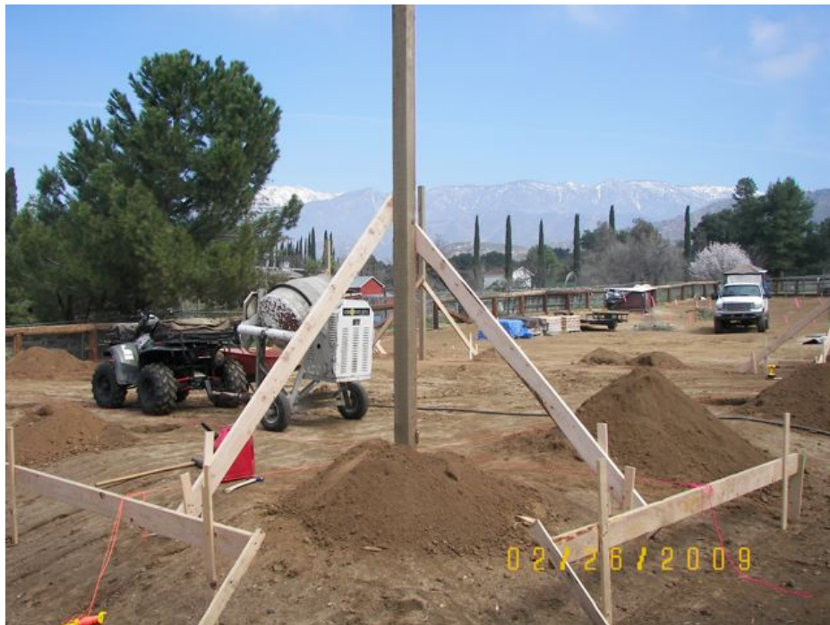
Photo above shows corner column in hole with batter boards in place.
